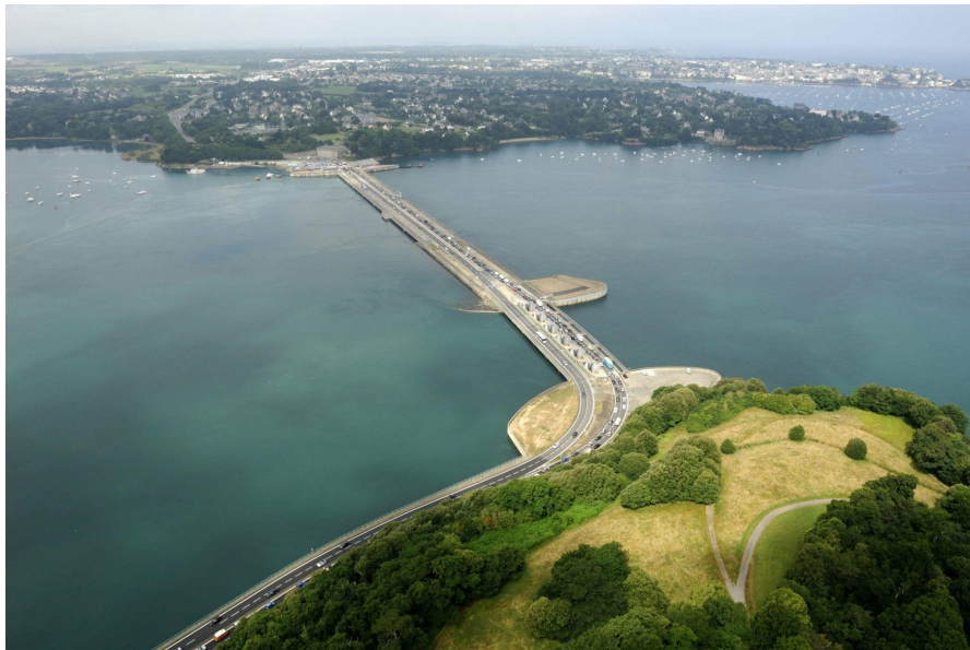
Figure 8. Tidal Range Technology: Rance Tidal Power Station in Brittany, France
