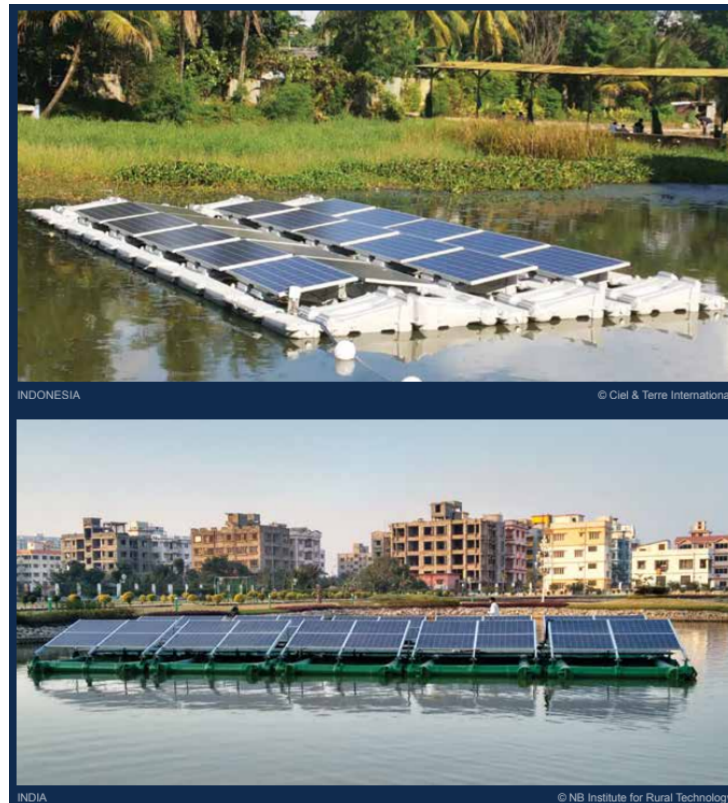
Figure 4. Marine Solar Technology
