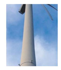
**DTBird® Collision Avoidance Module:** This module automatically emits warning sounds at birds flying in potential collision risk and discouraging sounds for birds flying in the high collision risk area. Adjustable to target species, wind turbine dimensions and local sound regulations. No energy production loss and useful for all bird species.
