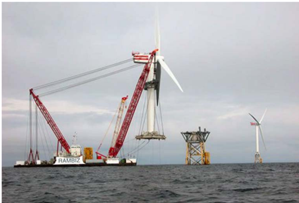
Figure 3.8: Beatrice Wind Turbines Installation
