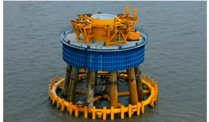
Fig. 2. High-Rise Structure Foundation (HRSF), Reprinted with permission from Xiao et al. (2020), Copyright 2020, Elsevier.
