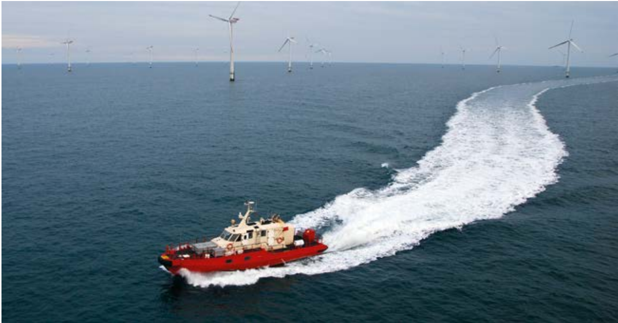
Service vessel leaving Horns Rev 1. PHOTO: VATTENFALL
