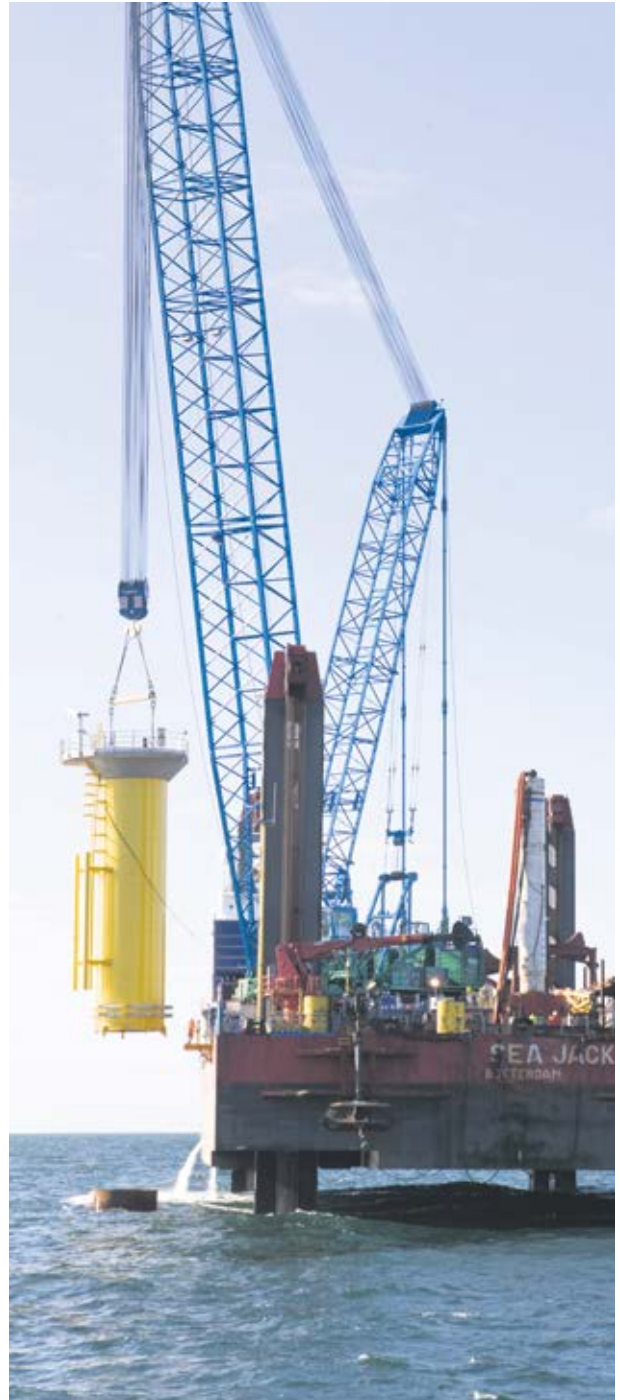
Construction of monopile foundations at Horns Rev 2.
