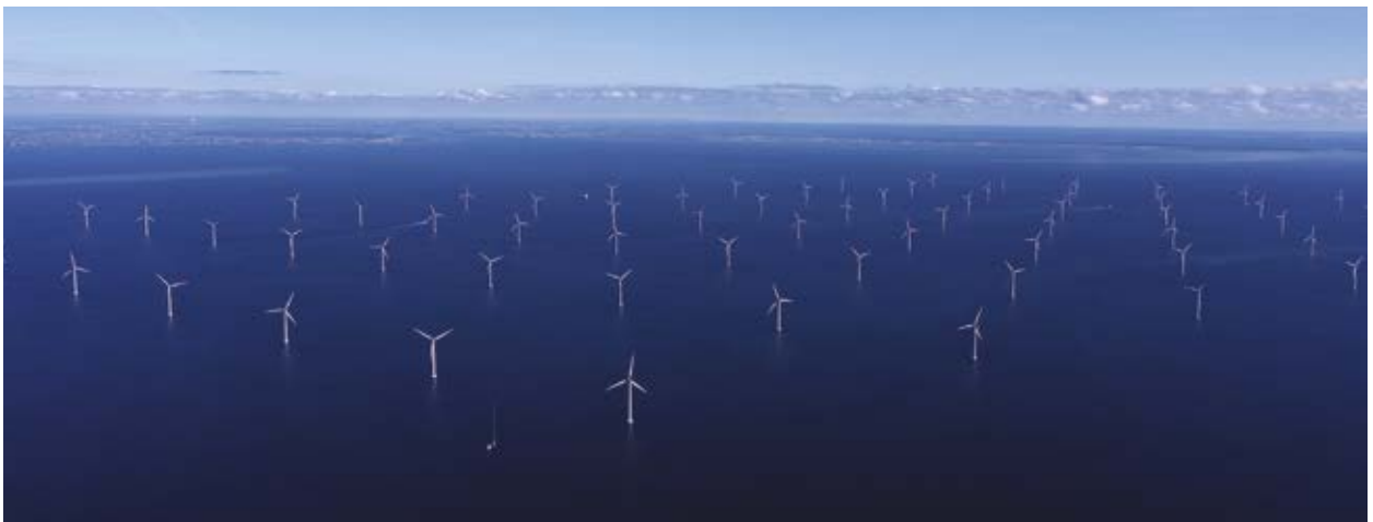
Nysted Offshore Wind Farm. PHOTO: NYSTED OFFSHORE WIND FARM
