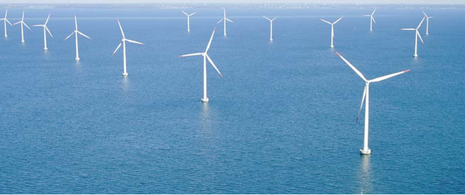
Nysted Offshore Wind Farm. PHOTO: NYSTED OFFSHORE WIND FARM
