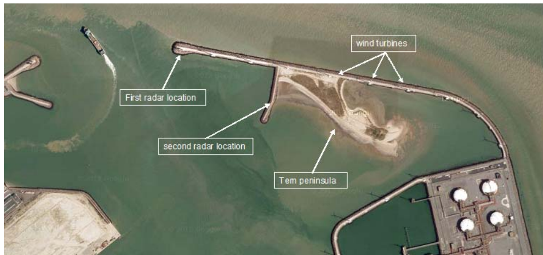
Figure 1. Radar test location in the port of Zeebrugge.
