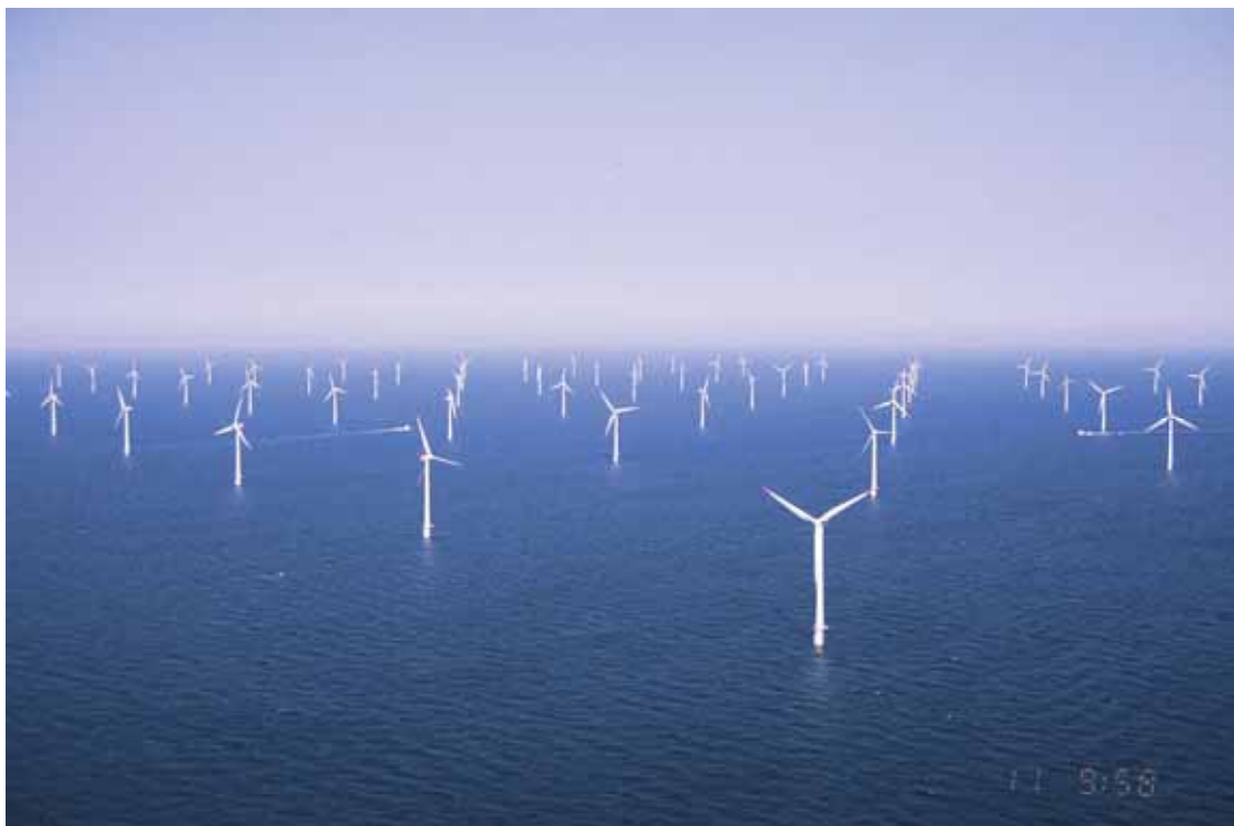
Figure 3. Aerial photo of Horns Rev Offshore Wind Farm. Photo: S. Tougaard.
