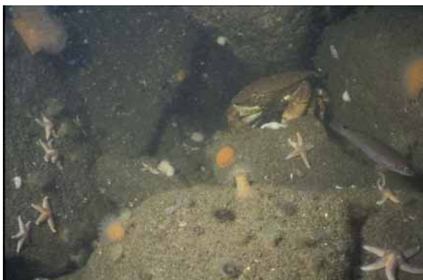
Figure 16. Scour protection boulders photographed in 2004 (two years after construction), with sea anemones, common starfish ( Asteria rubens ), an edible crab ( Cancer pagurus ) and Goldsinny-wrasse ( Ctenolabrus rupestris ). Photo: Bio/Consult A/S.
