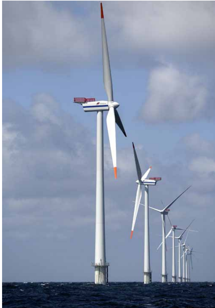
Figure 12 Turbines on Horns Reef seen from a point close to sea level (during maintenance, where turbines were stopped). Seastate 4-5 Beaufort. Photo: Vattenfall A/S.
