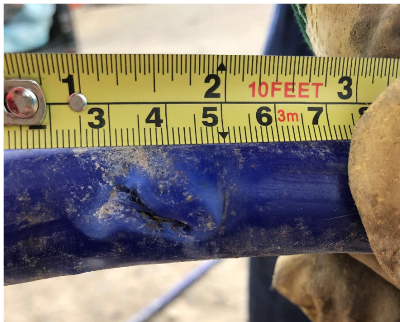
Figure 3. Damage to the umbilical cable connecting the HiCUP to the Turbine Support Structure (TSS).
