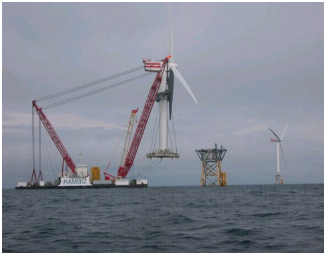
Figure O: Photograph of a heavy lift barge installing an offshore wind turbine. (Source: Saldis Salvage and Marine Contractors)
