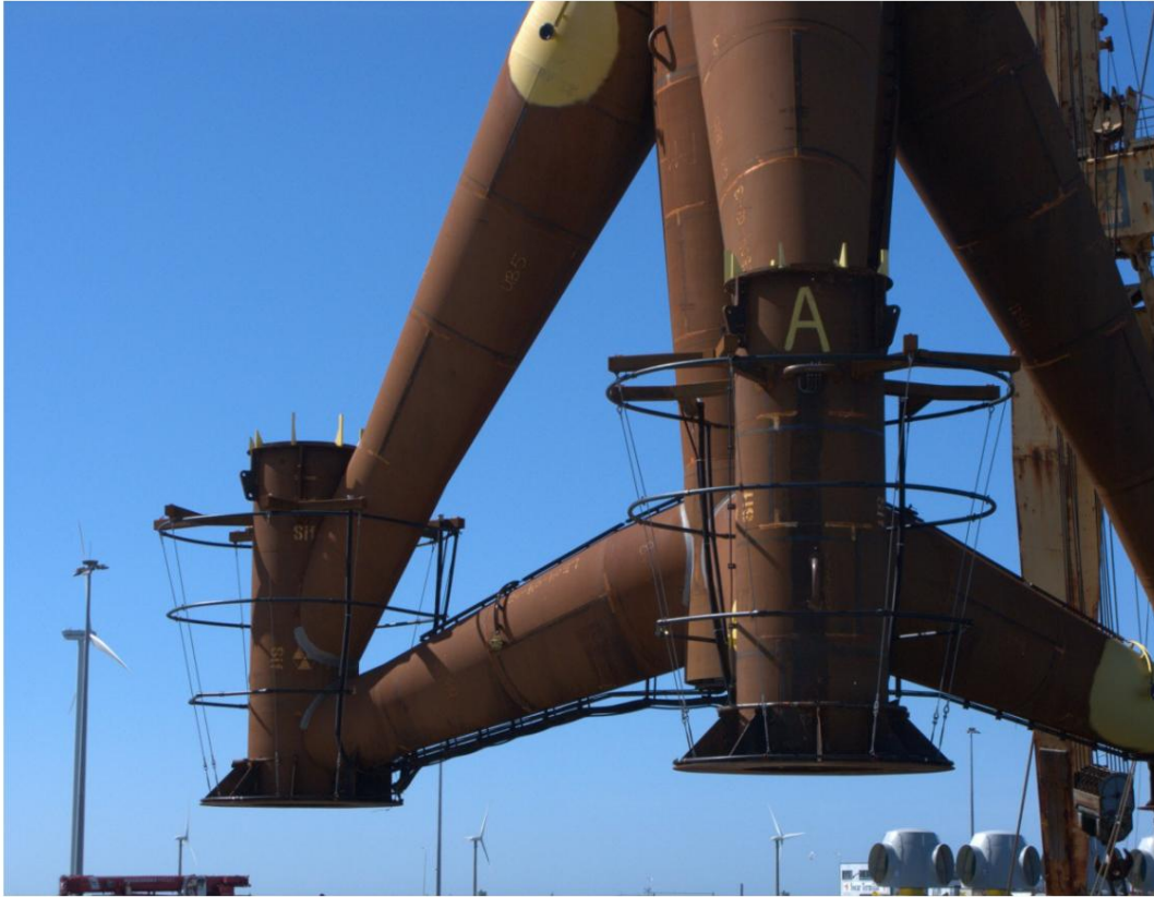
Figure 4-3: AV9 tripod foundation structure with two pre-assembled lower bubble curtain modules
