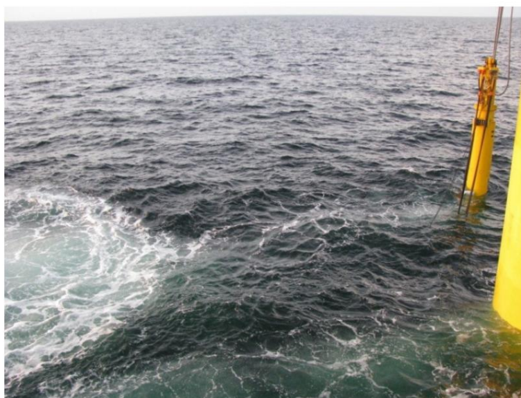
Fig. 5-25: Drift of the bubble curtain at 21:28 (CEST), on the right edge of the picture the main tube of the tripod, behind it the ram driving the northeast pile (ISD)
