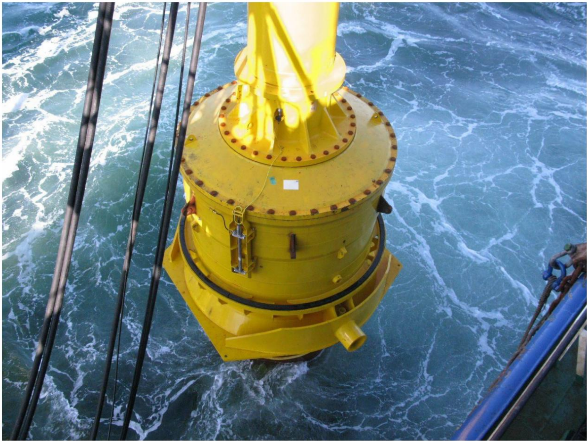
Fig. 4-5: Use of the "Little Bubble Curtain" noise reduction measure during the installation of a tripod in the alpha ventus test field
