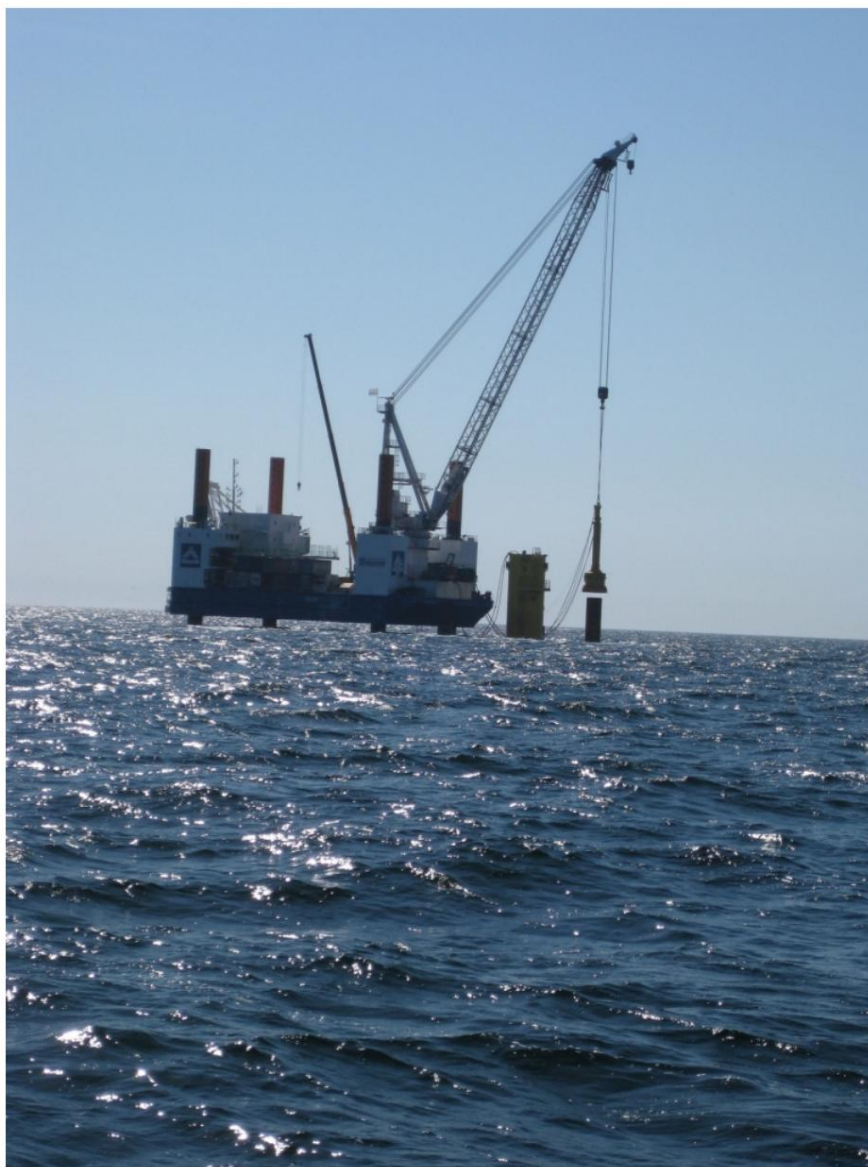
Fig. 5-2: Construction site seen from Baltic Taucher 2 (DEWI)
