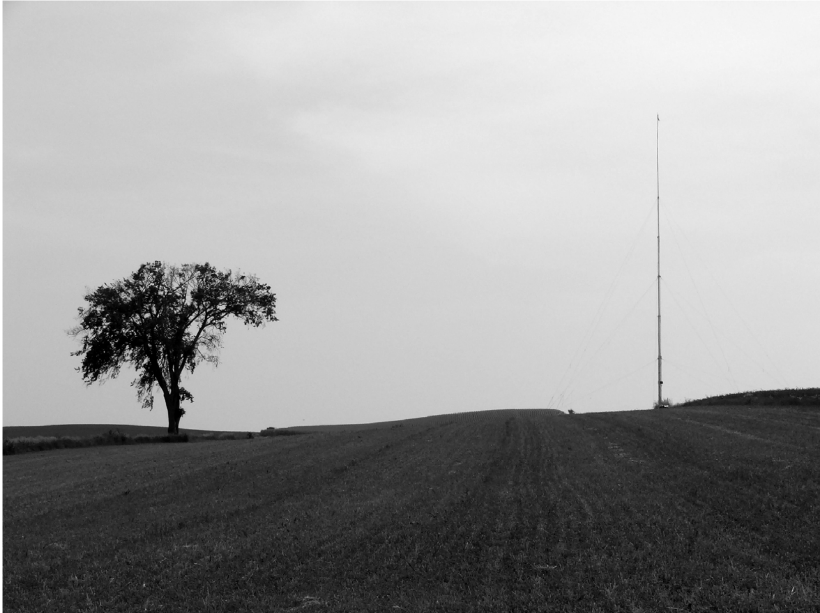
Figure 2. 22 m mobile tower used for mounting bat detector microphones at ground level (2 m) and 22 m above ground.
