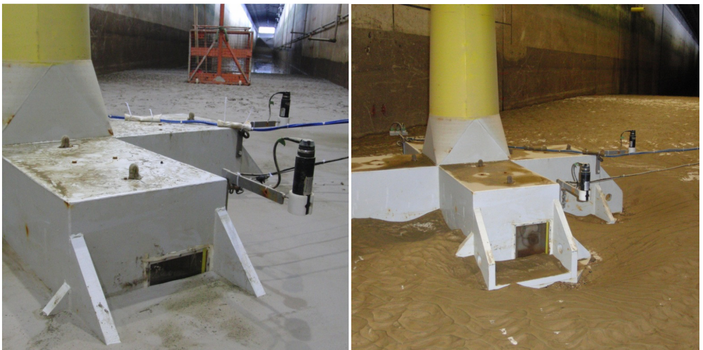
Figure 4-9: Echo sounder and underwater camera installation for point-wise, continuous scour recording in the GWK wave flume experiments.
