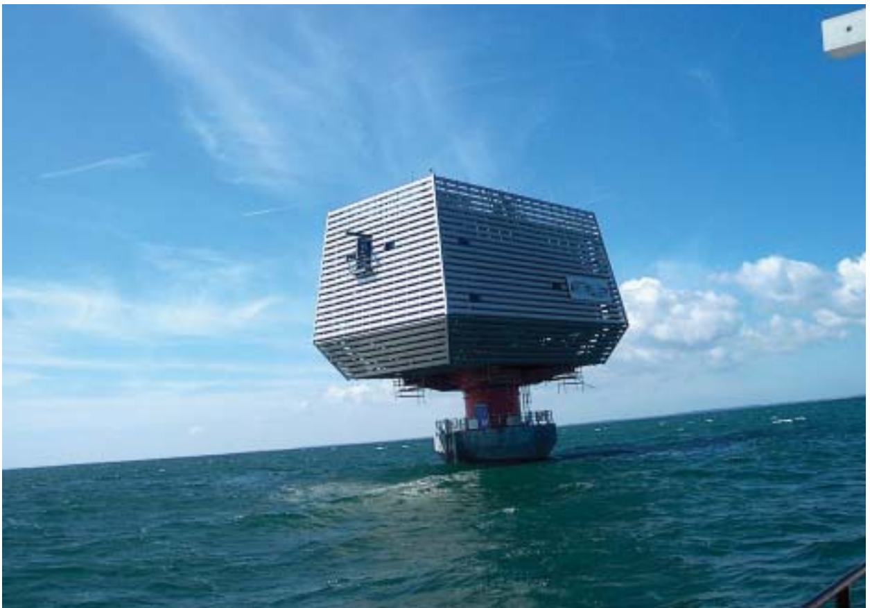
Transformer station, Nysted wind farm
