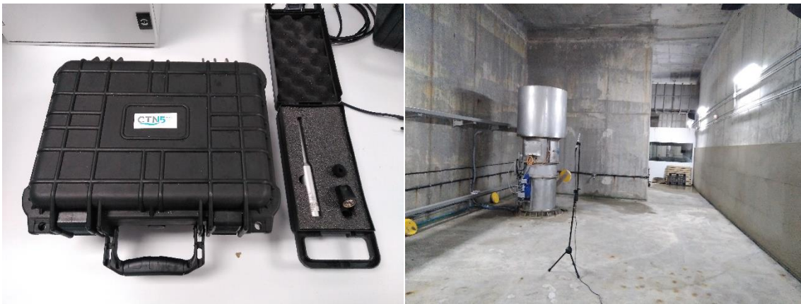
Figure 7. Left: Airborne acoustic monitoring system. Right: photograph of the microphone inside Mutriku Power Plant.
