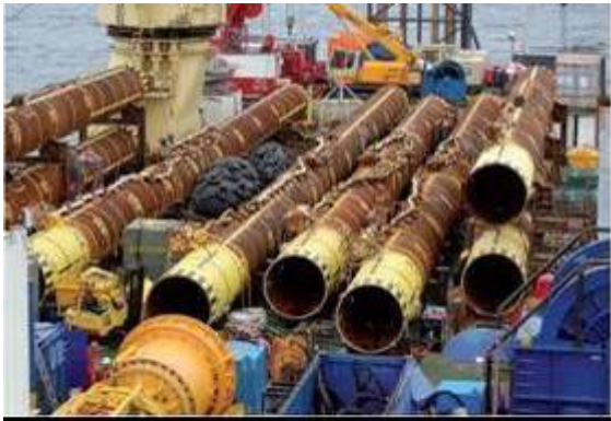
Figure 16 Multiple Mooring Piles Loaded for Transport
