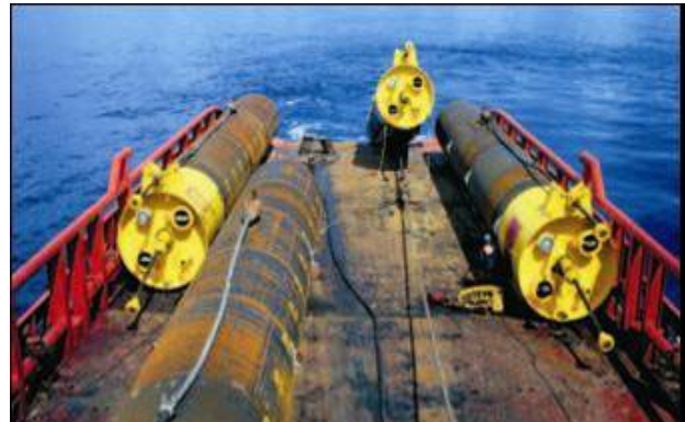
Figure 17 Multiple Suction Piles Installed from Single Vessel
