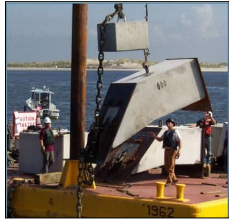
Figure 13 Enhanced Deadweight Anchor
