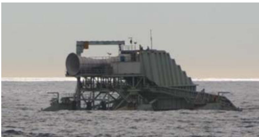
Figure 4. An oscillating water column device, developed by Oceanlinx (formerly Energetech, Australia)
