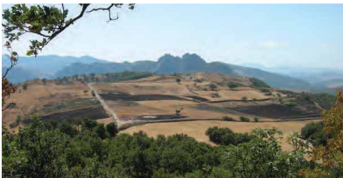
Italian wind farm construction site that has displaced red kites.
