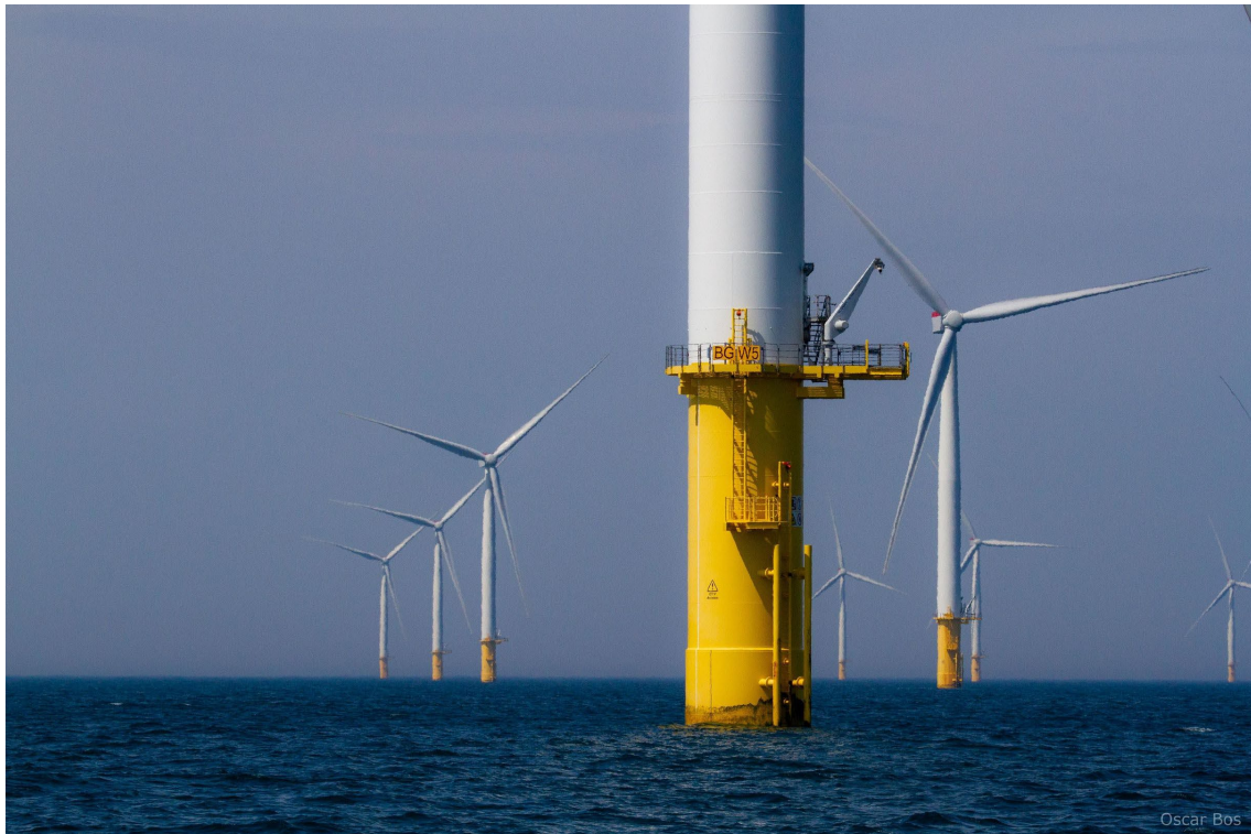
Figure 2. Turbine W5 in Gemini offshore windfarm.
