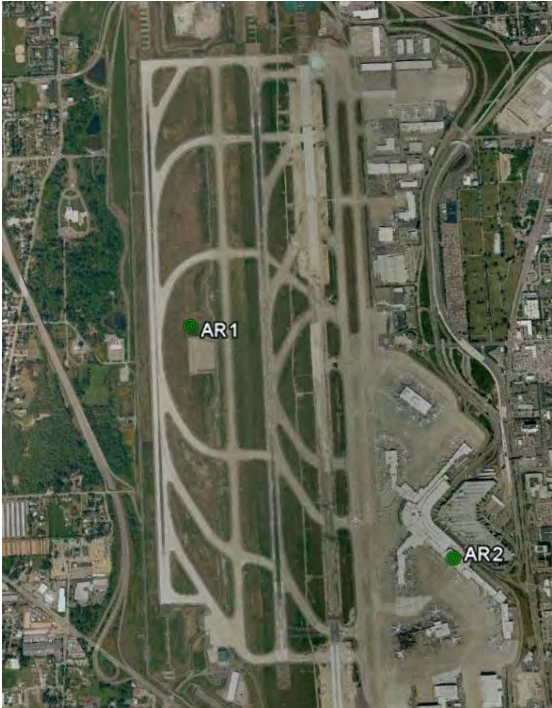
Figure 6-87. Locations of three avian radar systems operating at SEA. The AR-2 is comprised of two radars.
