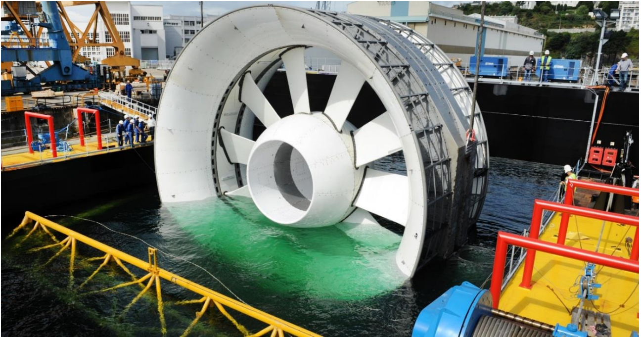
Figure 5.9: Open-Centre turbine and subsea base installed on barge in France, 2011 (OpenHydro)
