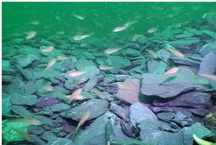
Figure 15 Barren rock dumped to fill scour pit and cover J-tube at Turbine 21. Photographer: F. Bunker
