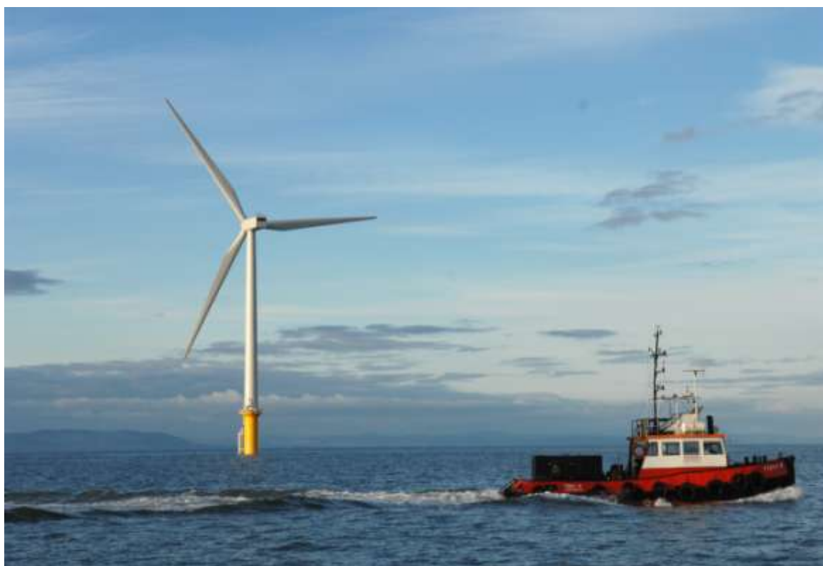
Figure 6: Maintenance vessel at the existing Burbo Bank offshore wind farm
