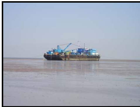
Figure 2 Photograph of the LM Construction barge aground at low water, after undertaking cabling works.
