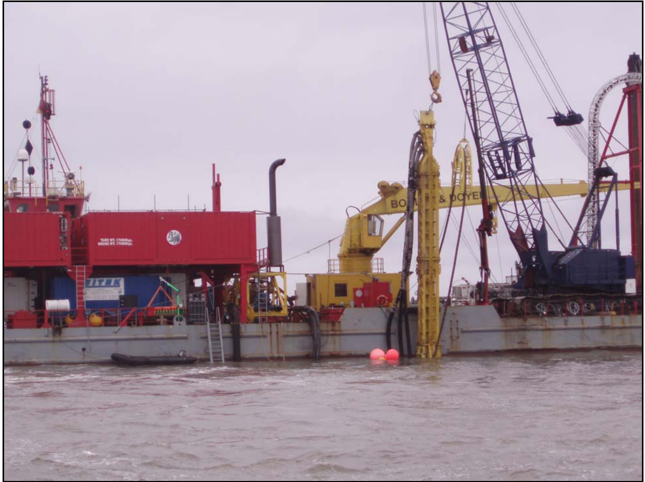
Plate 2. Burbo export cable installation in progress on 31 st August 2006.
