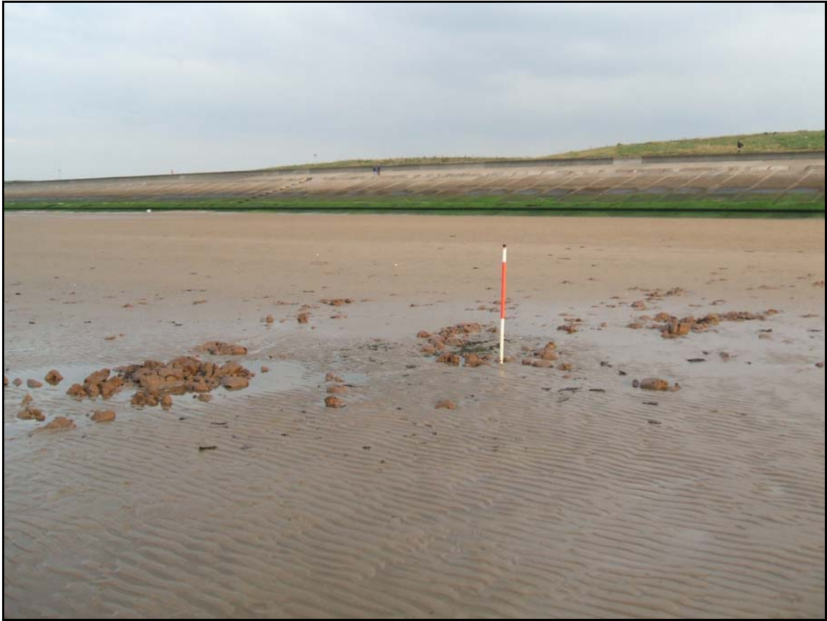
Figure 9. Site 31HDD 8 days after cable exposure and re-burial.
