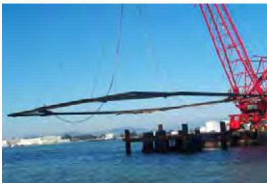
Figure I.9-4a Simple Air Bubble Ring Used during Driving of PIDP Pile 2
