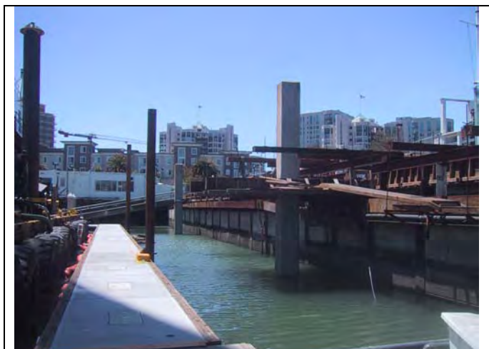
Figure I.5-5 24-Inch-Square Piles at Pier 40 – San Francisco, CA
