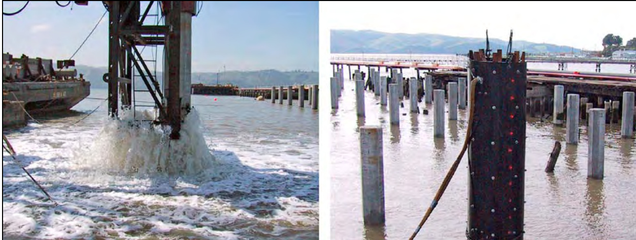
Figure 2-31. Simple Confined Air Bubble Curtain System
