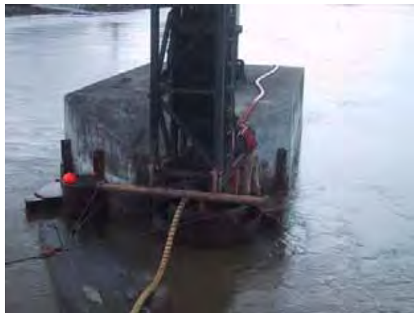
Figure I.11-2c Double-Walled Attenuator – Humboldt Bay Bridges, Eureka, CA
