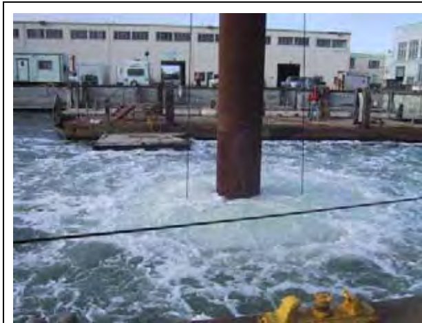
Figure I.3-26a Driving 40-Inch-Diameter Piles with Air Bubble Curtain in Alameda, CA
