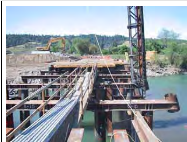
Figure I.3-17a Construction of the Temporary Trestle across the Russian River
