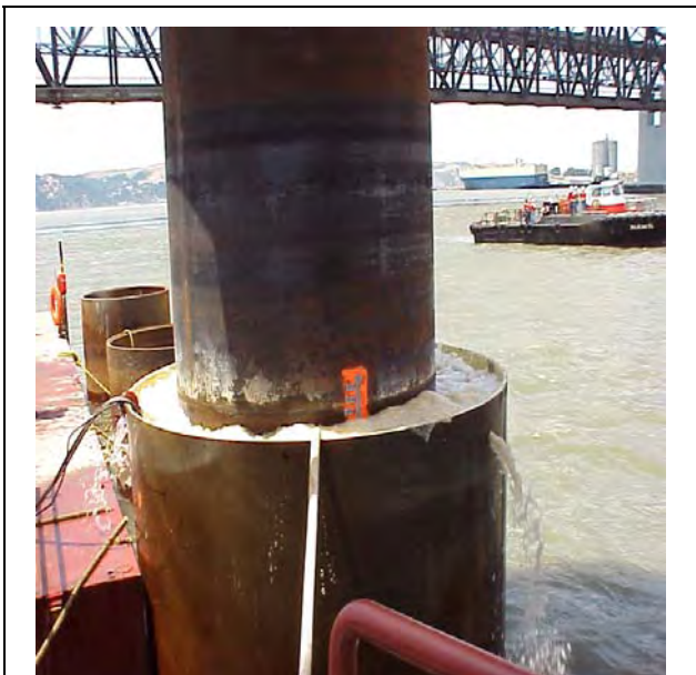
Figure I.8-4 Isolation Casing/Air Bubble Curtain System Tested for the Benicia-Martinez Bridge
