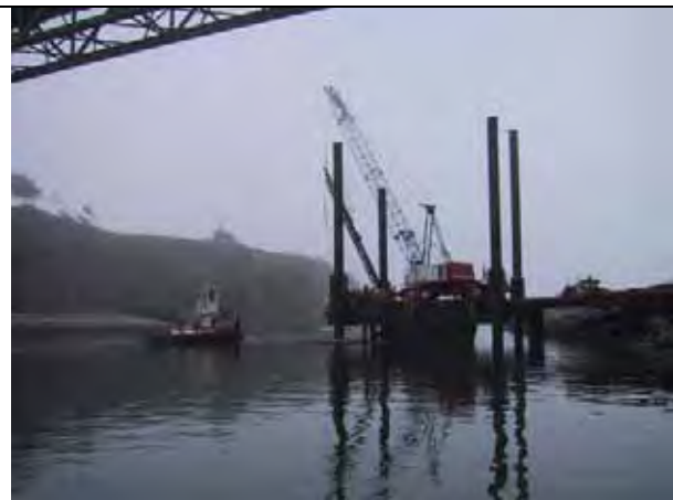
Figure I.4-1b Impact Driving of In-Water H-Type Piles
