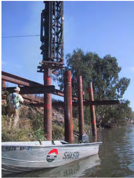
Figure I.3-7a Driving 20-Inch-Diameter Piles near Shore
