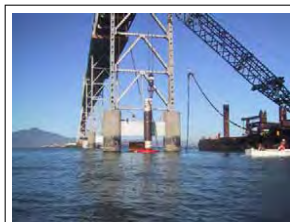
Figure I.10-12 150-Inch-Diameter CISS Pile Being Driven Underwater at the Richmond-San Rafael Bridge
