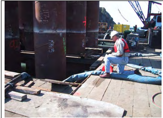
Figure I.3-1 CISS Piles Driven for the Noyo River Bridge Replacement Project
