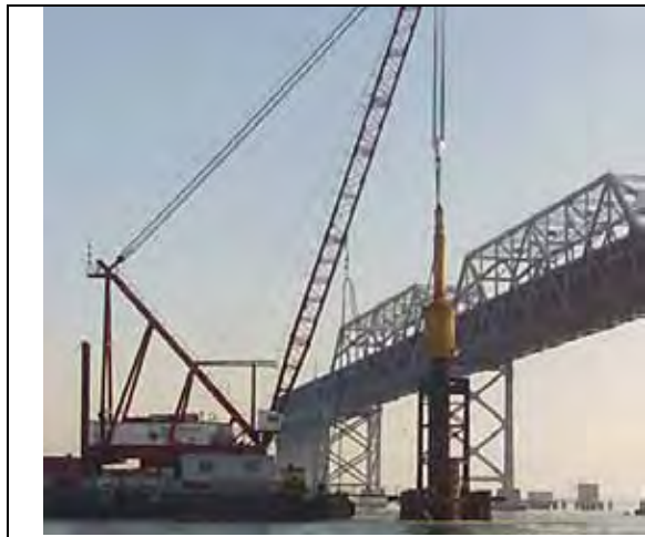
Figure I.9-3a Small Hydraulic Hammer (MHU500T) Used for Much of the Pile Driving
