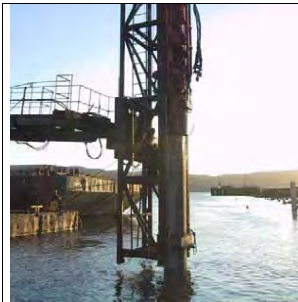
Figure I.5-4a 24-Inch Octagonal Piles Driven at Amports in Benicia, CA
