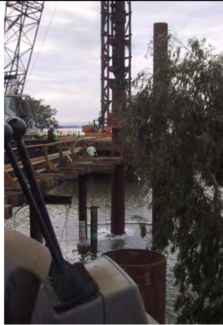
Figure I.3-7b Driving 36-Inch-Diameter Pile with Attenuation
