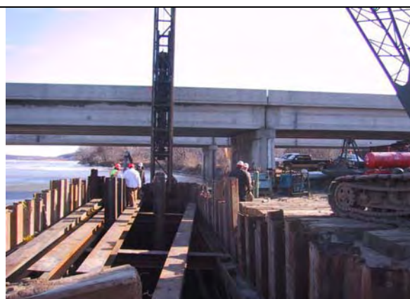
Figure I.4-5b Dewatered Cofferdam Excavated below Water Level
