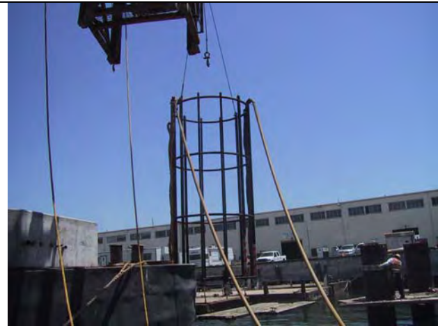
Figure I.3-26b Air Bubble Curtain Used at Bay Ship and Yacht, Alameda, CA
