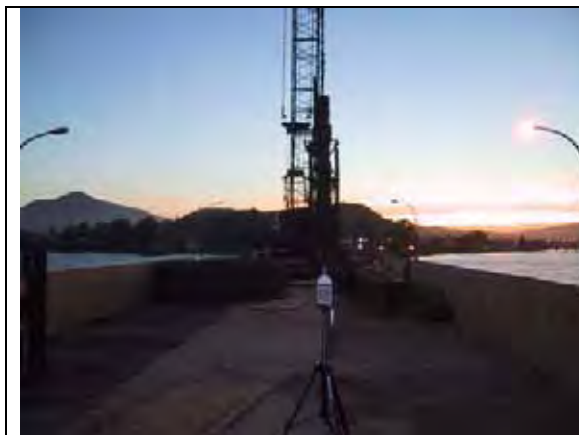
Figure I.10-4 30-Inch-Diameter Pile Being Driven for Temporary Trestle at Richmond-San Rafael Bridge
