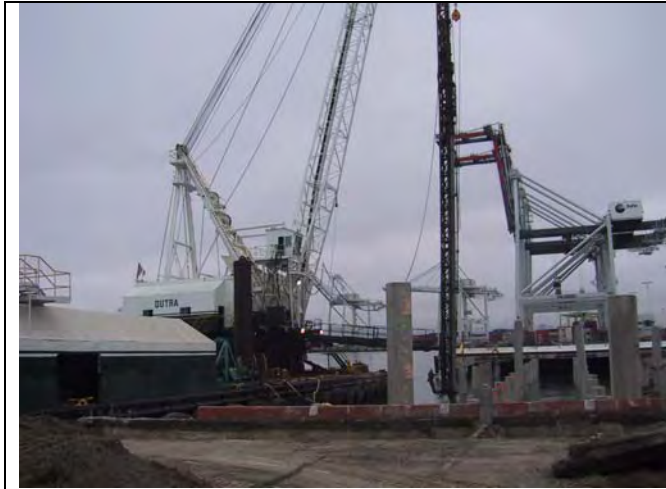
Figure I.5-10 Driving of 24-Inch Octagonal Piles at Berth 32, Port of Oakland, CA
