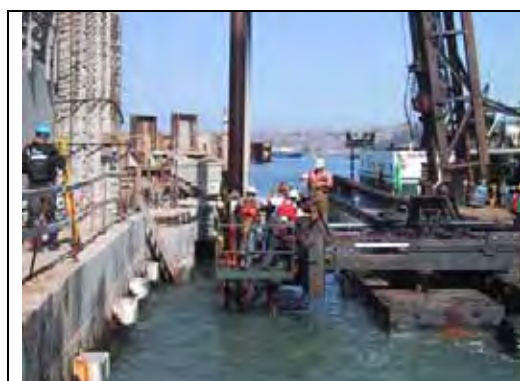
Figure I.10-2 14-Inch-Diameter Pile Being Driven next to Pier at Richmond-San Rafael Bridge
