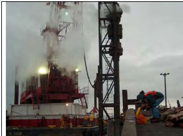
Figure I.5-1a Driving of 16-Inch-Square Piles
