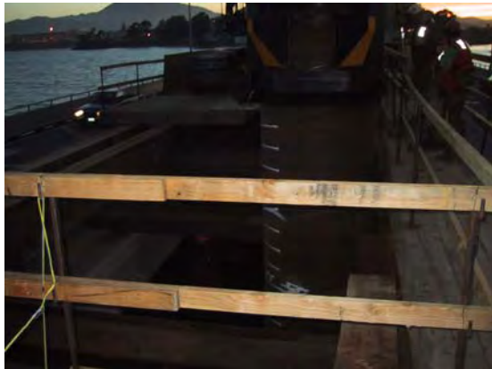
Figure I.10-7 66-Inch-Diameter CIDH Pile Being Driven at Richmond-San Rafael Bridge
