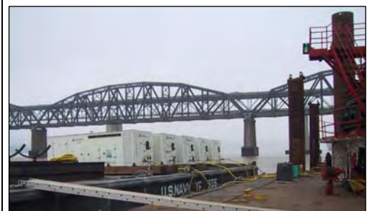
Figure I.8-6 Air Bubble Curtain Tree System Used at the Benicia-Martinez Bridge
