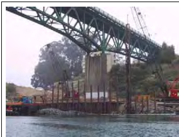
Figure I.4-1a Impact Driving of On-Shore H-Type Piles
