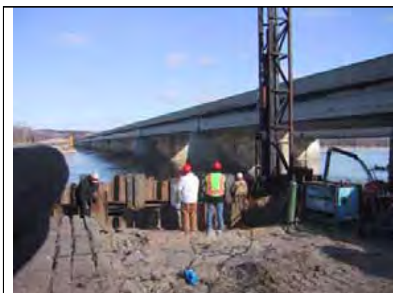
Figure I.4-5a H-Type Pile Driving at the Platte River in Nebraska
