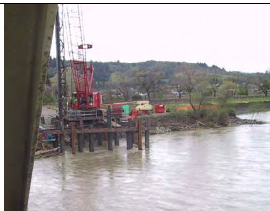
Figure I.3-18b Attempting to Stab Pile through Casing (Noise Control) on West Bank
