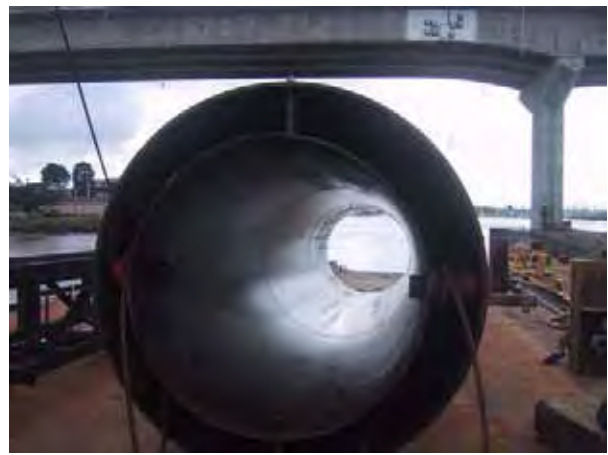
Figure I.11-2b Unconfined Air Bubble Curtain Used at Slack Tide – Humboldt Bay Bridges, Eureka, CA
