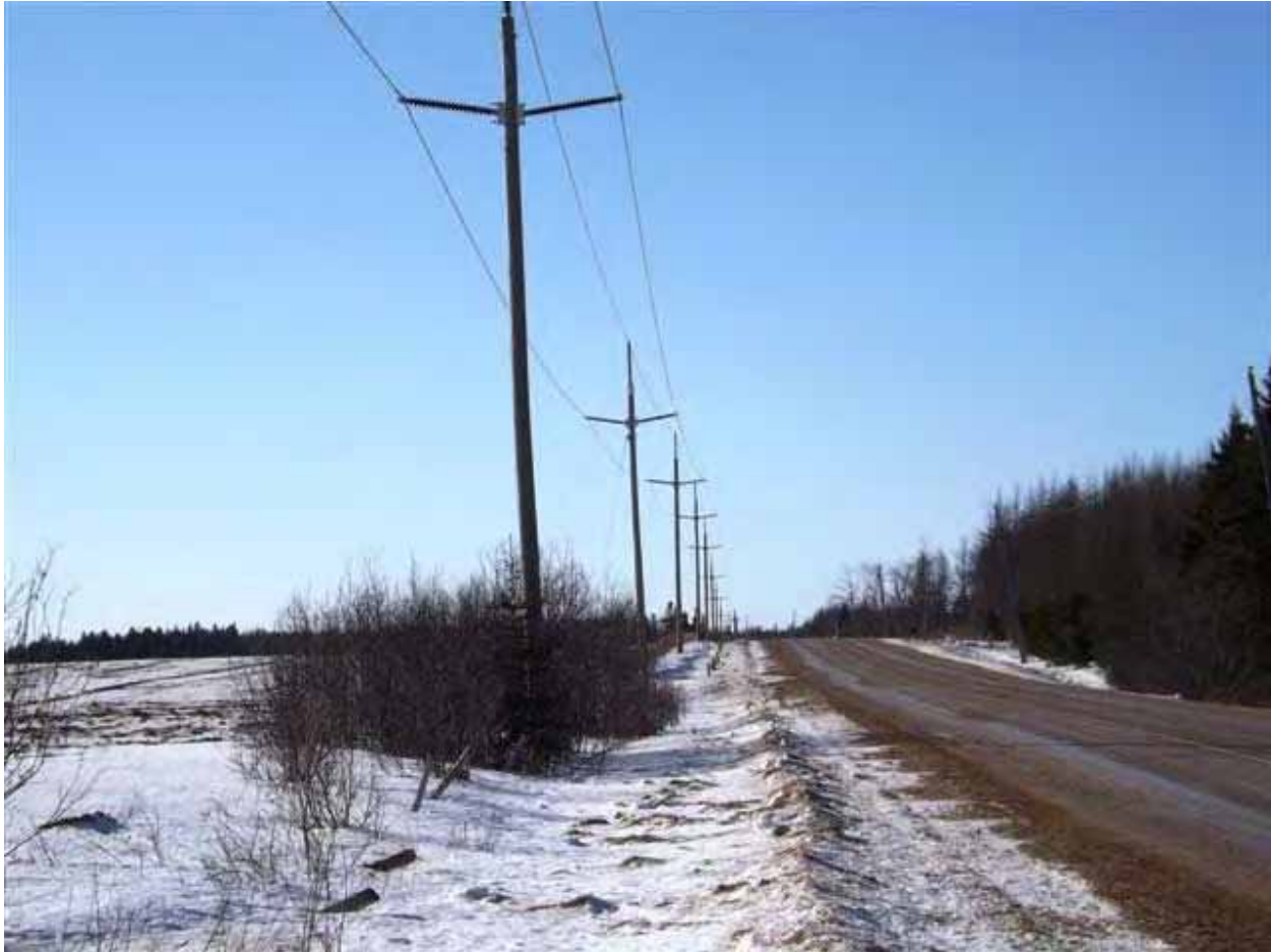
Figure 2.7 Typical Transmission Line Construction
