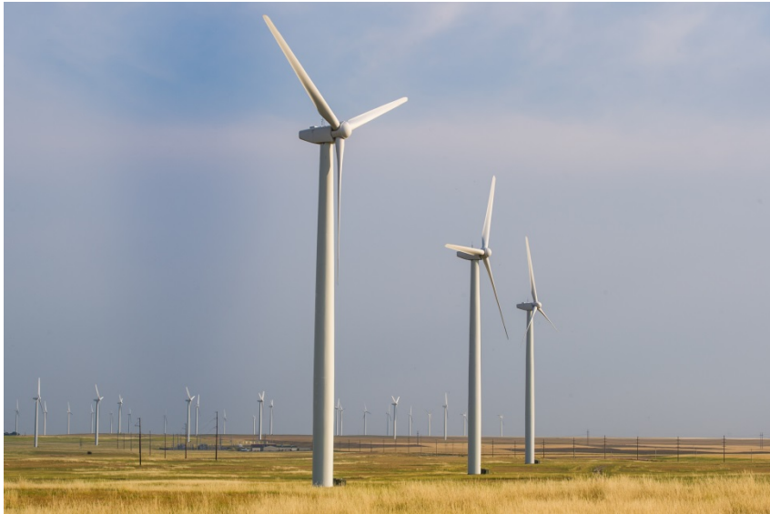
Cedar Creek Wind Farm in Grover, Colorado. Photo by Dennis Schroeder, NREL 30590
