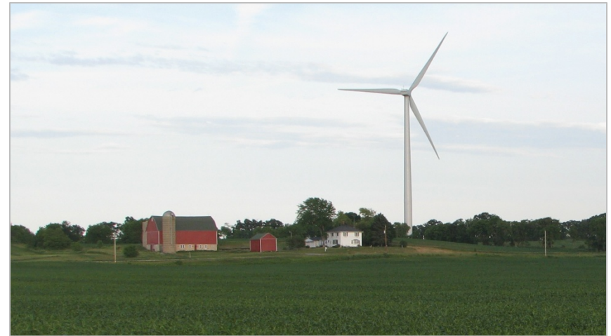
Forward Wind Energy Center in Fond du Lac and Dodge Counties, Wisconsin. Photo by Ruth Baranowski, NREL 21208
