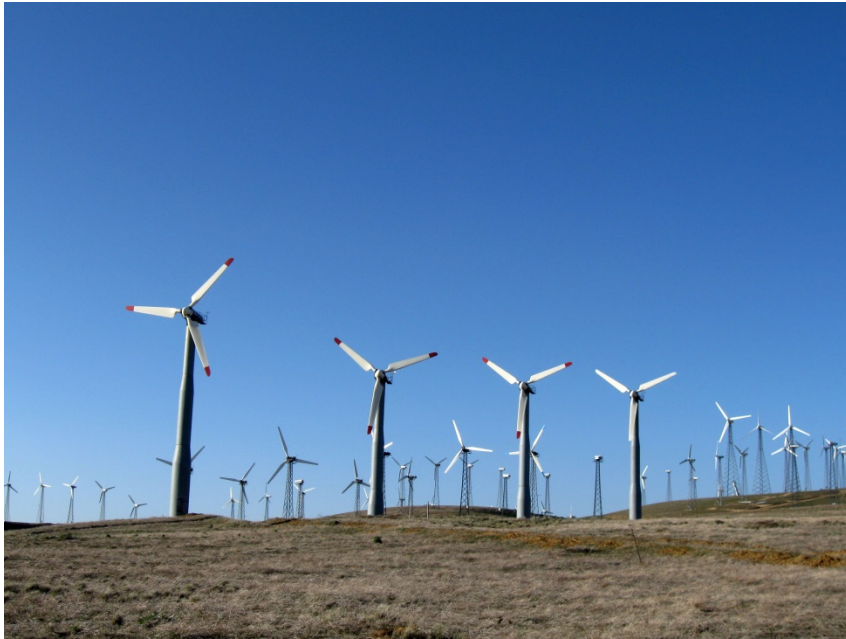
705-megawatt Tehachapi Pass Wind Farm. Photo by David Hicks, NREL 18455-C
