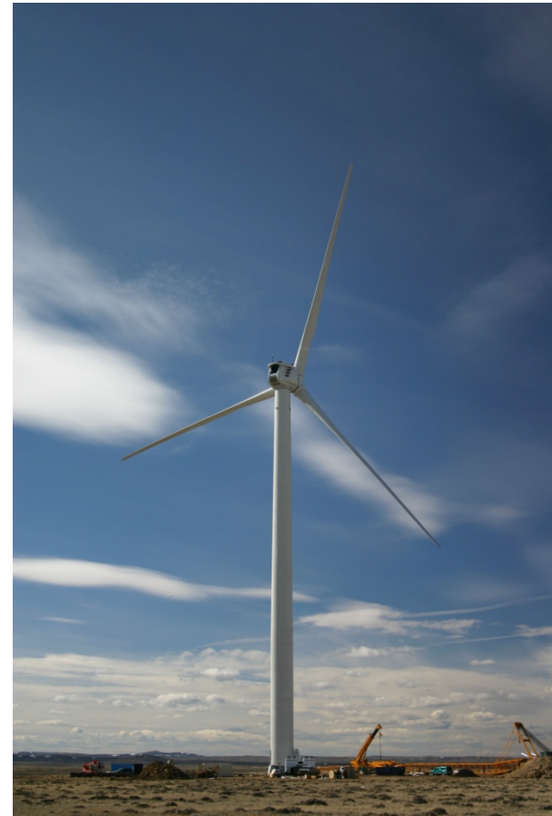
Clipper 2.5-MW wind turbine with a 93-meter diameter. Photo by Alan Laxson, NREL 13886
