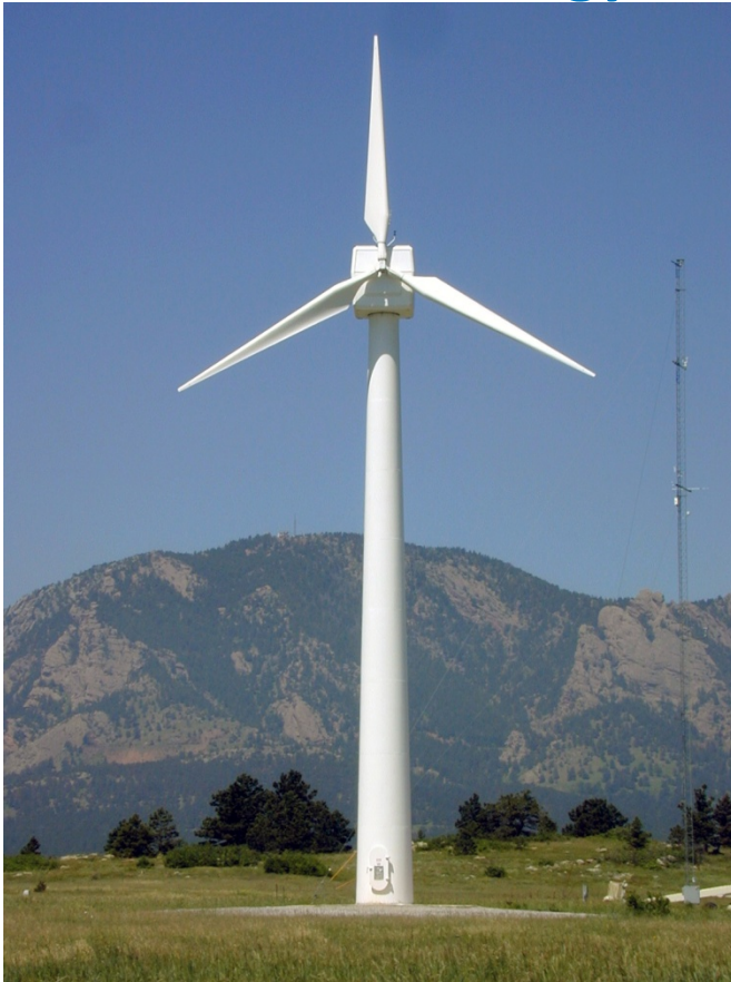
19-meter diameter blades on a 100-kW turbine. Photo by Lee Jay Fingersh, NREL 16392
