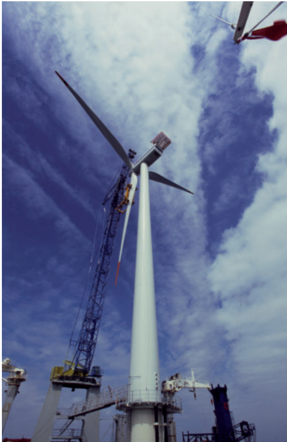
Mounting of turbine tower at Horns Rev.
