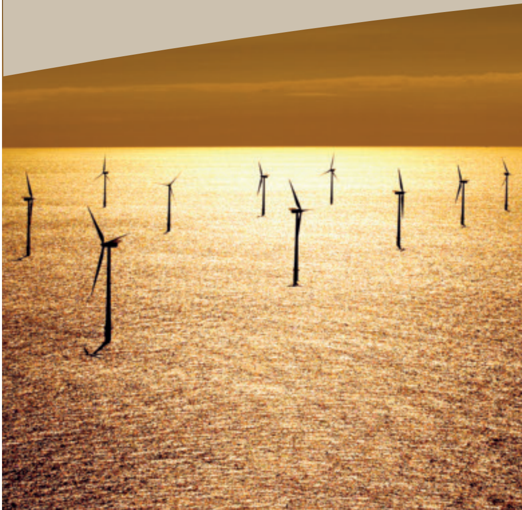
Horns Rev Offshore Wind Farm.
