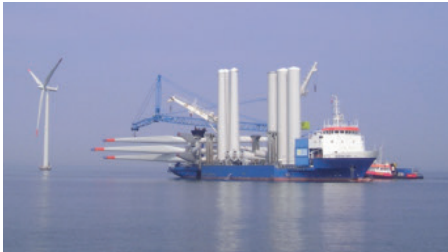
The ship Ocean Ady in front of the first wind turbine at Nysted. Turbines no. 2, 3 and 4 lie ready on deck.
