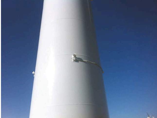
Figure 5. DTBird Detection Module HD cameras installed on the WTG tower. Two to eight HD cameras can be installed per wind turbine. (photo from leaflet on www.dtbird.com )
