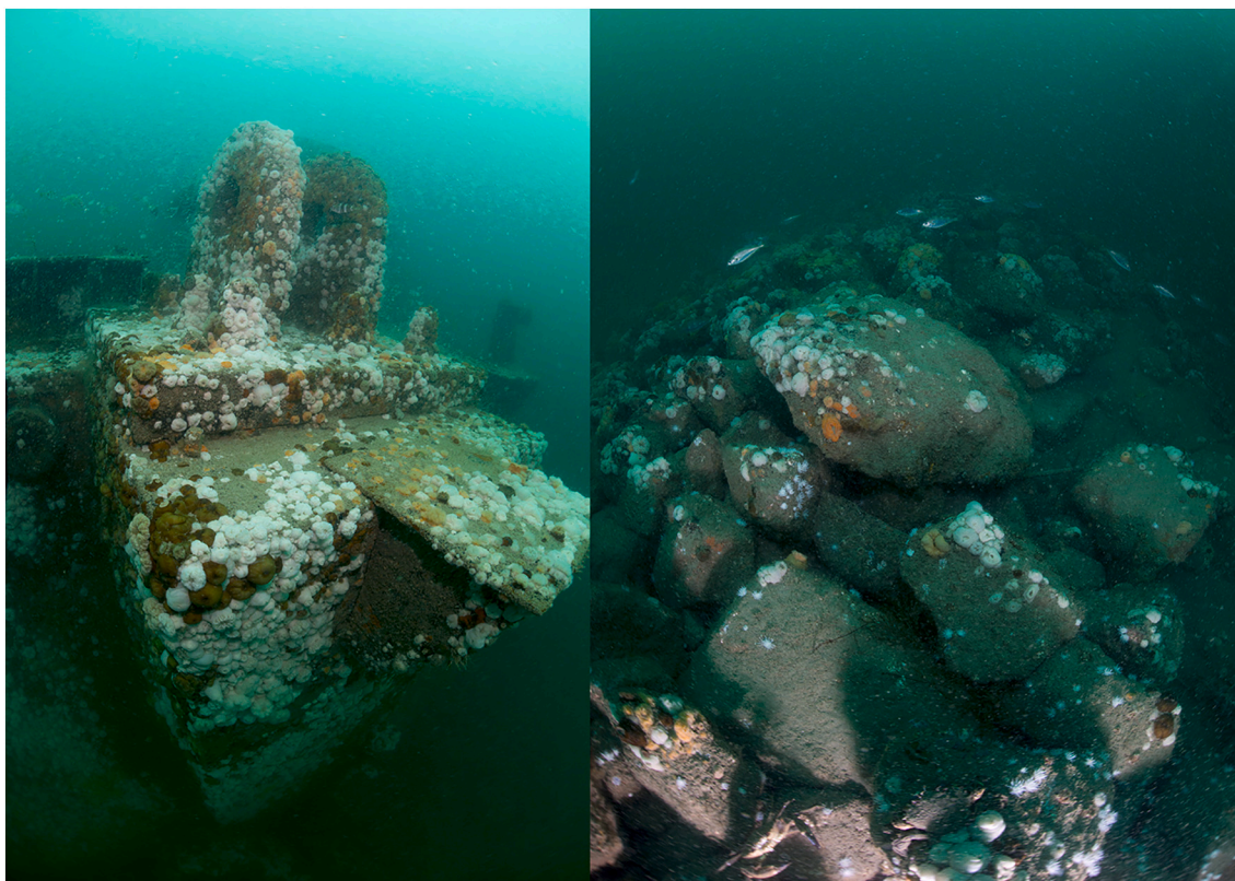
Fig. 3. In situ impression of the Halfweg GBS and rock dump. Under water photographs of: left: a detail of the GBS showing one of the lifting points and surrounding concrete substrate; right: overview of the rock dump surrounding the GBS. Photos by Udo van Dongen (Bureau Waardenburg b.v.).
