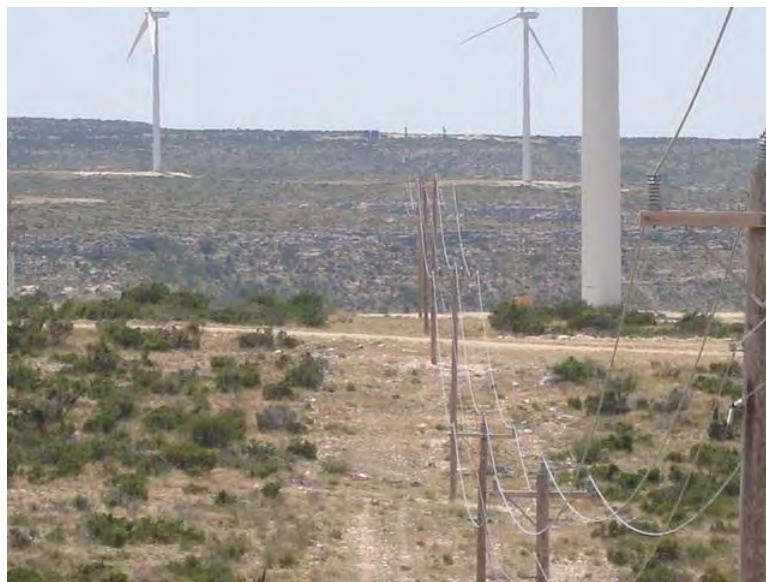
Figure 2-9 Typical Structures for Aboveground Collector Lines
