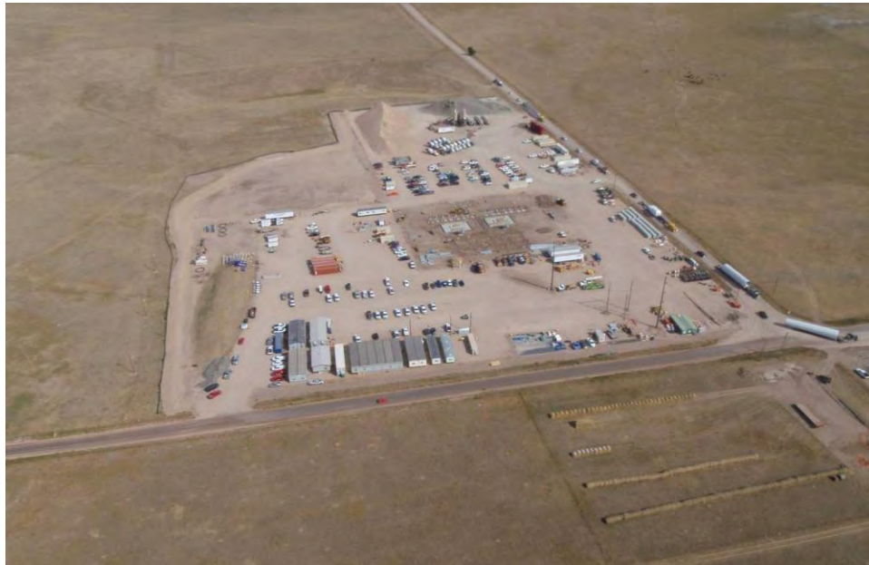
Figure 2-1 Typical Construction Laydown Area
