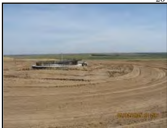
Figure 2.3-8. Typical WTG Spread Foundation During Construction
