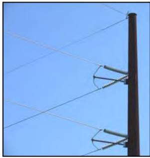
Typical Conductor Connections
