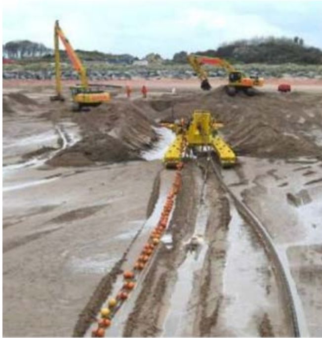
Figure 5.14: Tidal Zone Cable Plough Trenching
