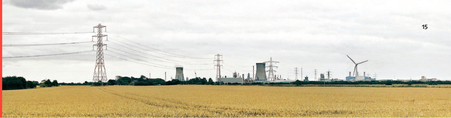
Photomontage – viewpoint from Westfield Farm looking south towards the proposed substation (infrastructure between two cooling towers).
