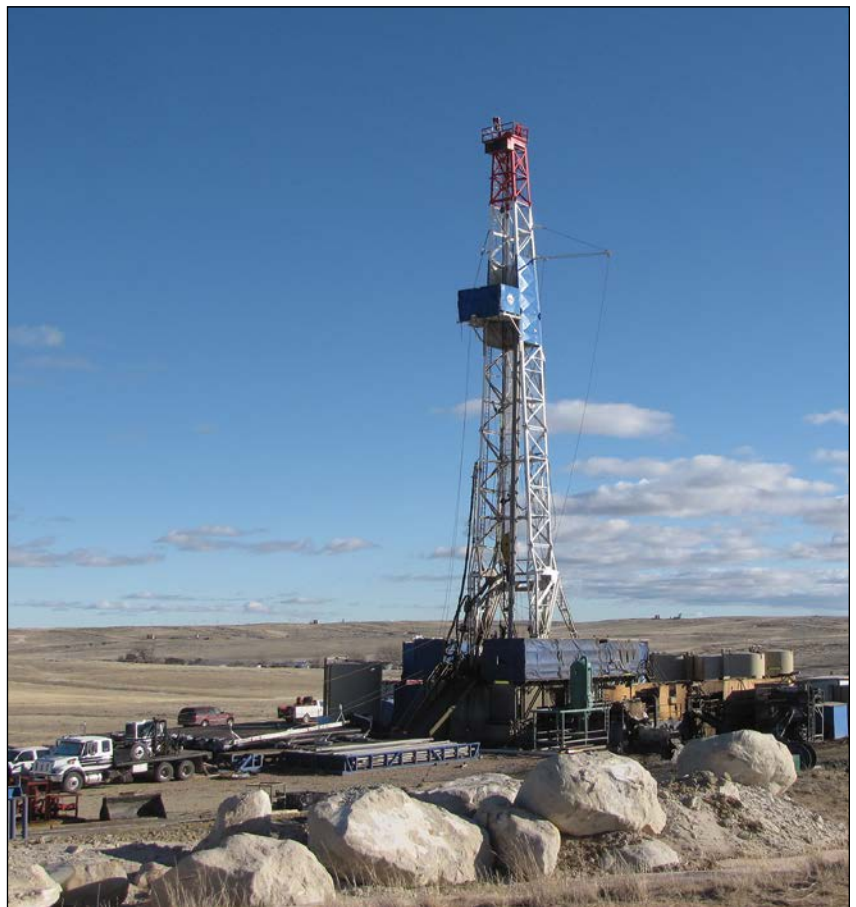
This oil rig in Wyoming is an example of long directional drilling, which can limit the amount of surface disturbance due to the rig’s long reach. Photograph by Bureau of Land Management.
