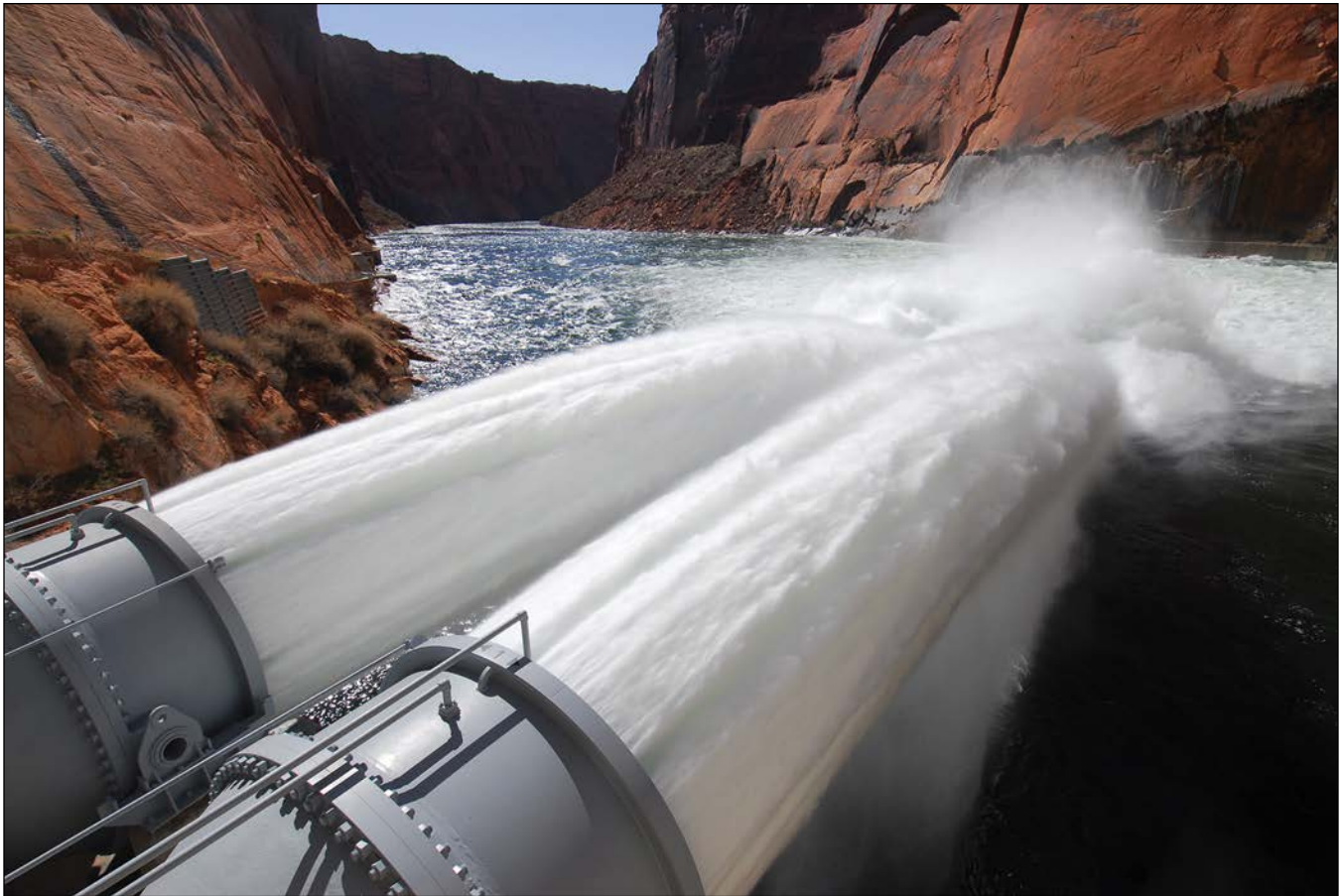
Photograph by U.S. Geological Survey.
