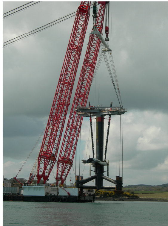
Plate 1.2: SeaGen quadropile lowered into position.
