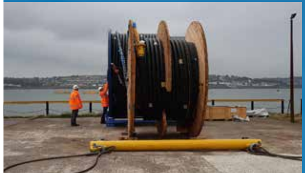
mWave cable delivered to the dockside at Pembroke Dock Port
