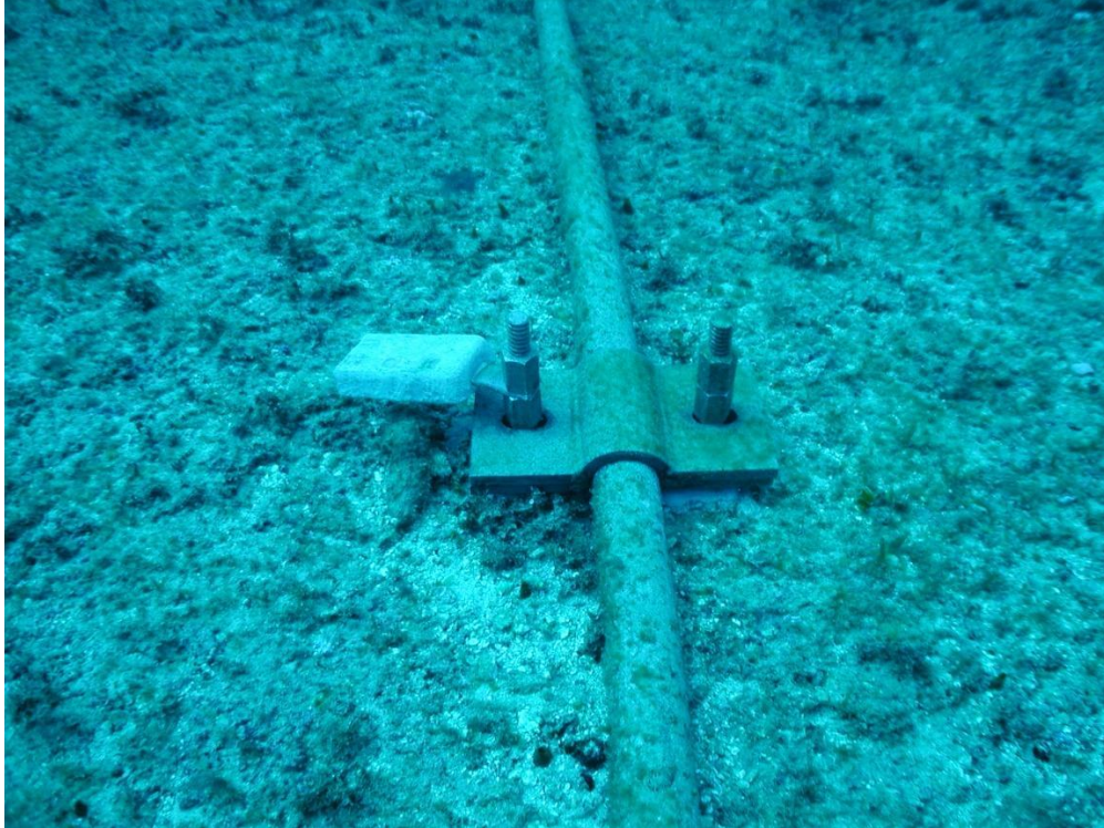
Figure 14. Power cable with anchor bolt at 50 ft in March 2005
