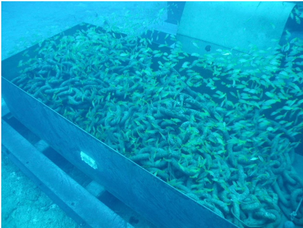
Figure 4. Anchoring/mooring base after installation (Winter 2004)
