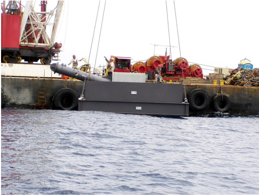
Figure 3. Anchor/mooring base being installed (Fall 2003). Note ballast chain to the right
