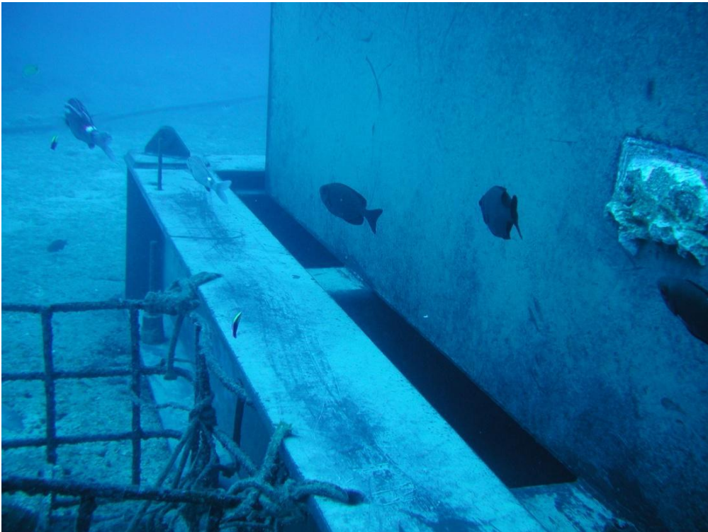
Figure 9. Mooring base in early 2004. Note the minimal fouling
