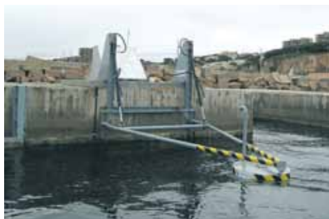
1/4 scale Abencis Seapower prototype installed in Sant Feliu de Guíxols (Mediterranean Sea)
