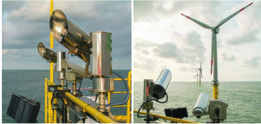
Figure 6 Daylight camera and thermal imaging camera installed on the transformer station outside the Alpha Ventus wind farm. Cameras are positioned in such a way as to monitor the Rotor Swept Zone of the turbine (images taken from Hill et al., 2014).
