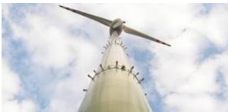
Figure 18 B-finder system installed onshore (images taken from Przybycin et al., 2019).
