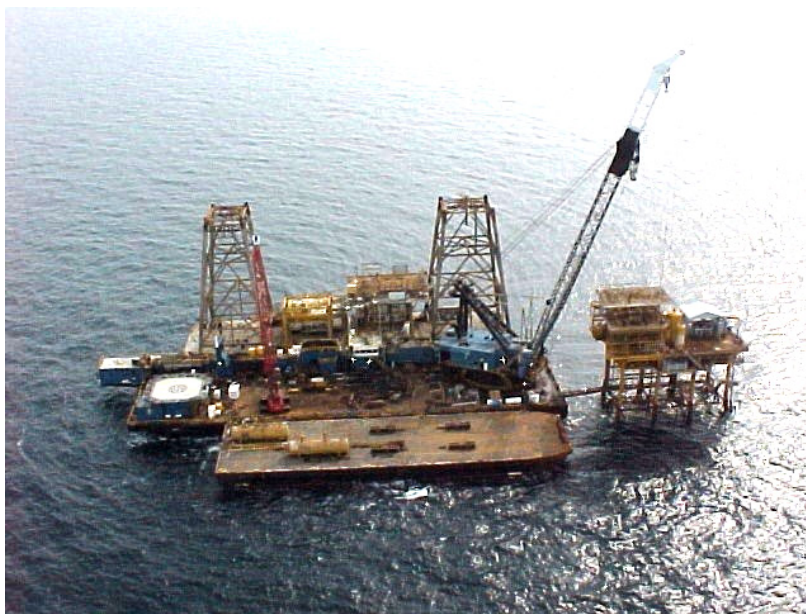
Figure 9 - Fugro Derrick Barge
