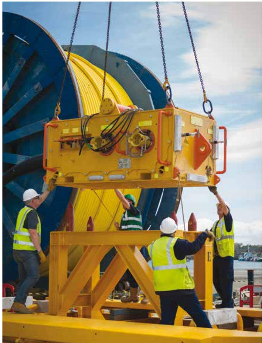
Image: JDR Cables
