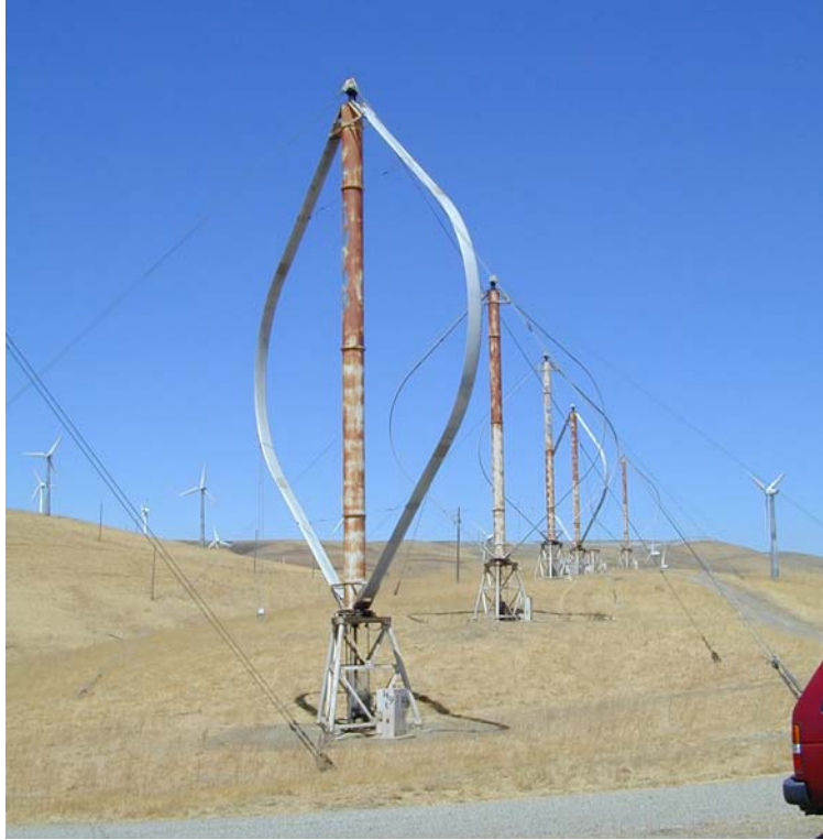
Photo 1. Flowind F-17 vertical axis wind turbines in the Altamont Pass Wind Resource Area prior to replacement in the Diablo Winds Energy Project.
