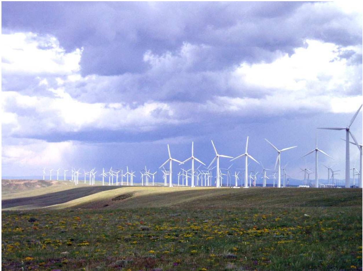
Footnote Creek Rim wind facility, Arlington, WY
