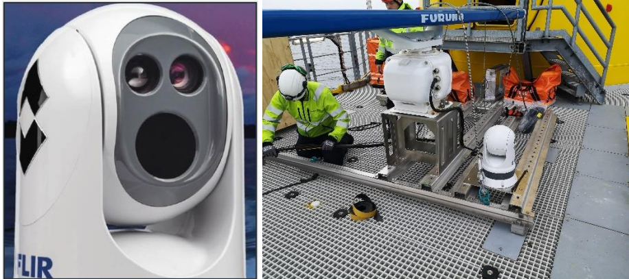
Figure 3-5 FLIR M400 camera, showing installation process at EOWDC
