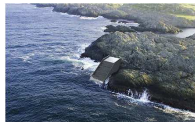
Figure 1: SSG pilot plant in Kvitsøy island, Norway [39].
