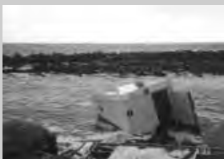
Public restrooms after 1999 storm at Ocean Shores. Photo - Brian Voigt
