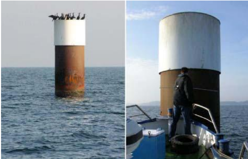
Fig. 1. The test pile in the vicinity of Travemünde. The white cover is intended to make it more visible to shipping and is removed for pile-driving experiments (photos from autumn 2005).
