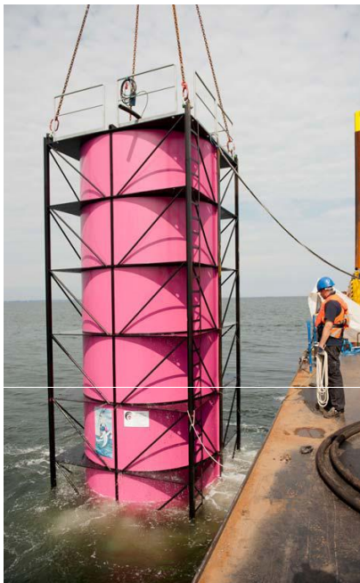
Figure 23: BeKa jacket during installation (photo: Patrice Kunte)
