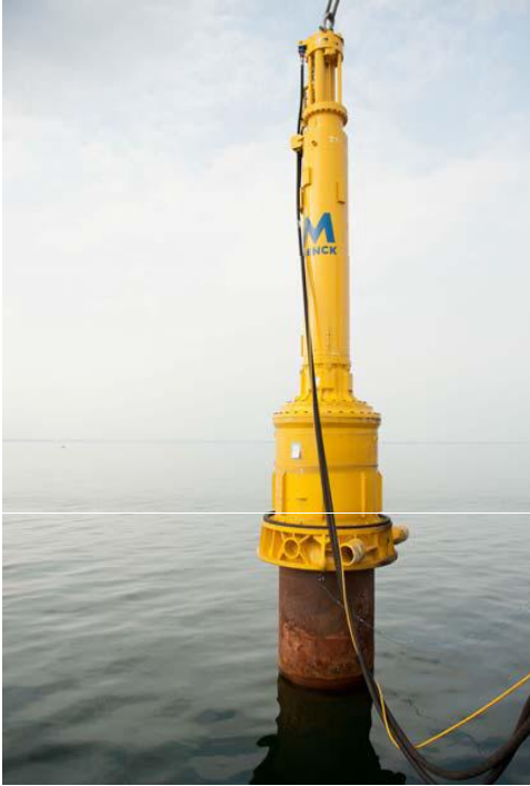
Figure 7: Hammer placed on the pile (photo: Patrice Kunte)
