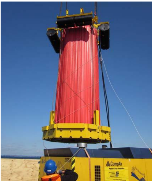
Figure 14: Menck fire hose system being lifted off the deck of the work platform (left) and during installation at the pile (right) (photo: Patrice Kunte)
