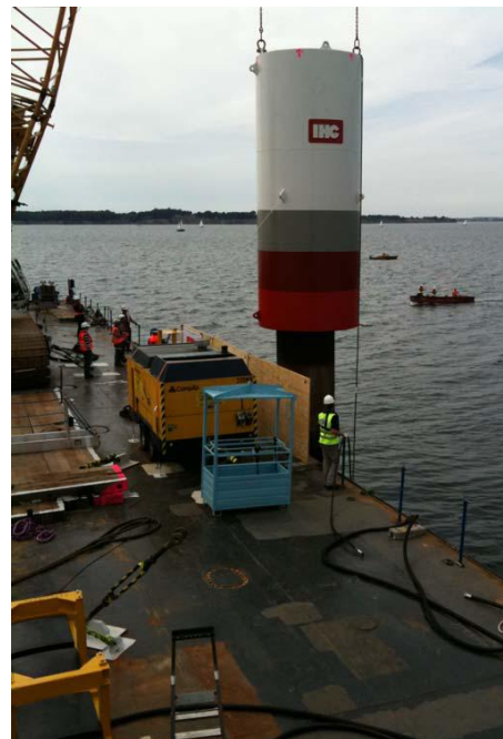
Figure 12: IHC NMS during installation (photo: Patrice Kunte)
