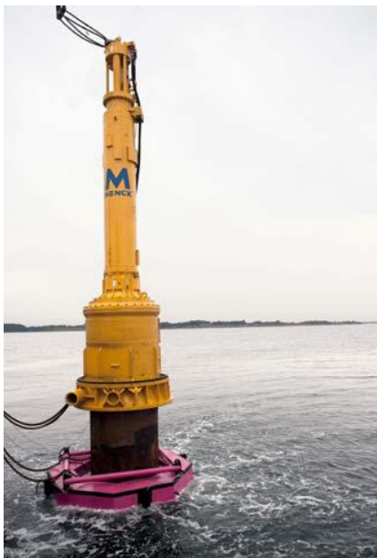
Figure 20: Weyres little bubble curtain in operation (photo: Patrice Kunte)
