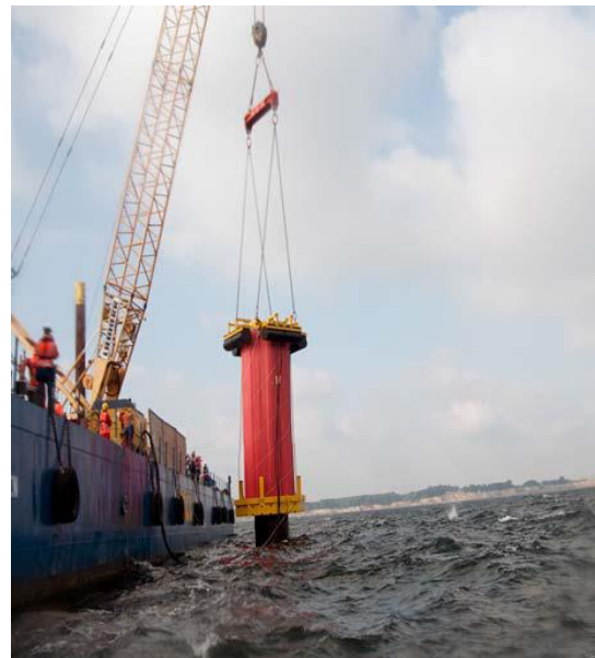
Figure 14: Menck fire hose system being lifted off the deck of the work platform (left) and during installation at the pile (right) (photo: Patrice Kunte)
